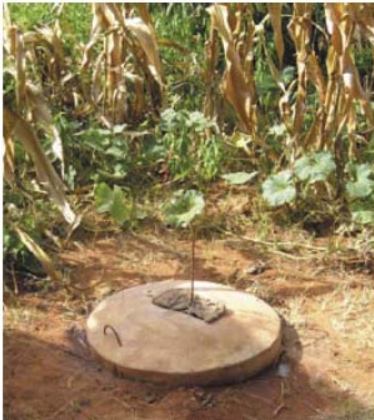
A child-size "arbor-loo" latrine provides children with a safe sanitation solution. Photo: © Water For People / by Kate Harawa
