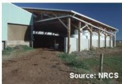
Water run-off control with the use of a gutter system at the Fenk Dairy, Tillamook, Oregon. In the public domain.
