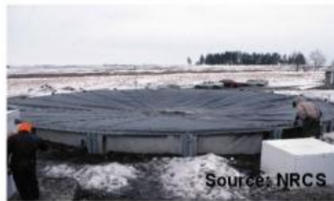
Methane recovery unit in Story County, Iowa In the public domain.
