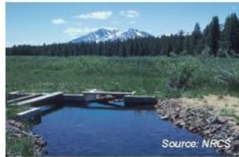
Diversion structure is part of a well planned irrigation system. ID
