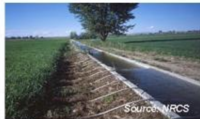
Surface irrigation system using siphon tubes , Idaho
